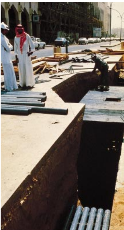
Pipe laying and installation of a distribution vault for an urban telecom system in Saudi Arabia.
