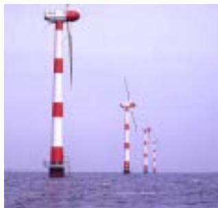
The near-shore wind turbine park, Lely, owned by Energie Noord West, consists of four NedWind40 turbines with a combined power of 2MW.
