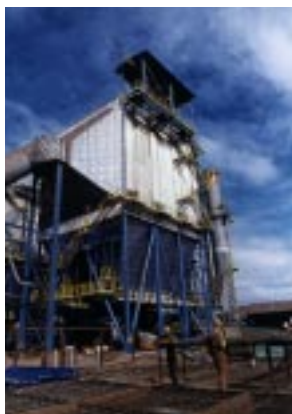
One of six electrostatic precipitators – huge anti-pollution devices which filter the air at the sinter plants
